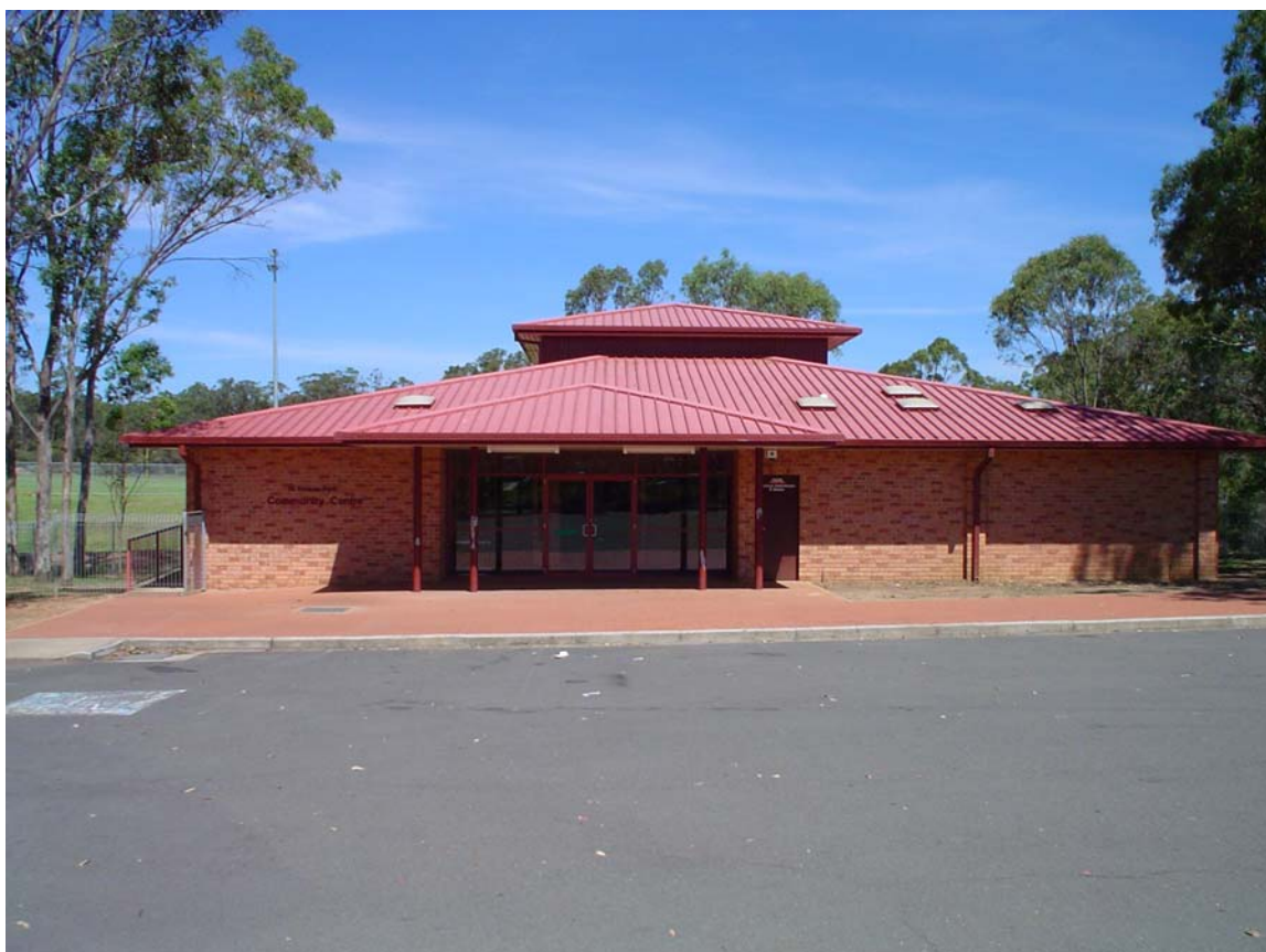
Figure 3: St Helen's Park Community Centre
